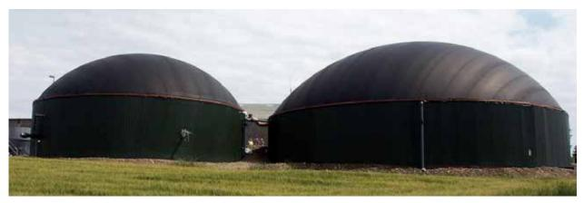
Figure 5.5 Anaerobic Digestion can be used to convert slurry into organic fertiliser, while the waste gas can be collected and used as a fuel. Picture from Irish Independent
